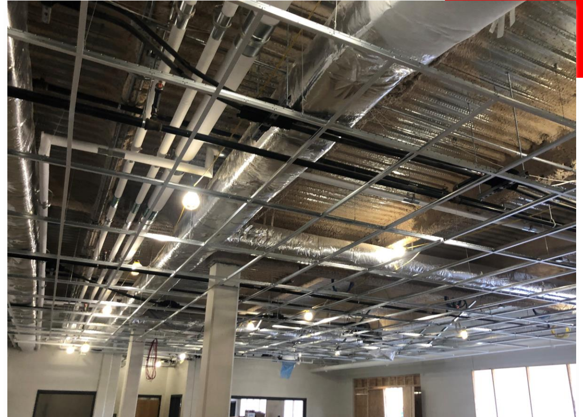
ACT Grid Completed First Floor of New Addition
